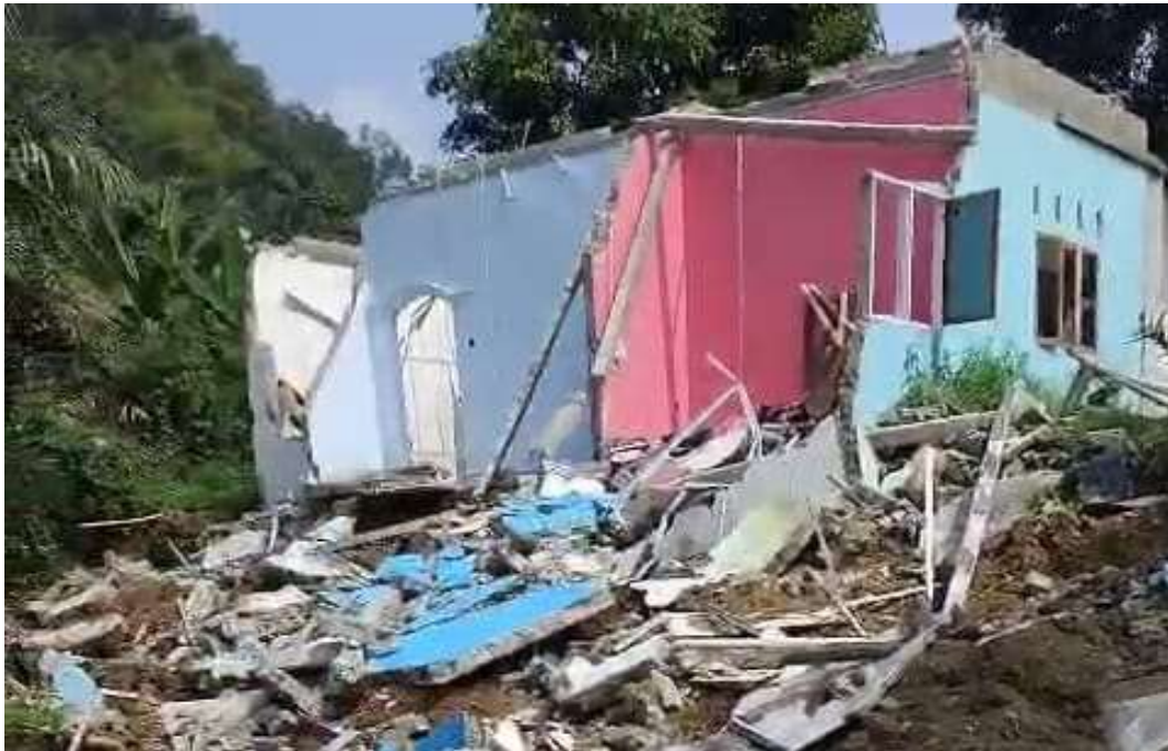
Figure 1. Destroyed Houses in Pasirmunjul Sukatani Village (Source: PDPI Document)
