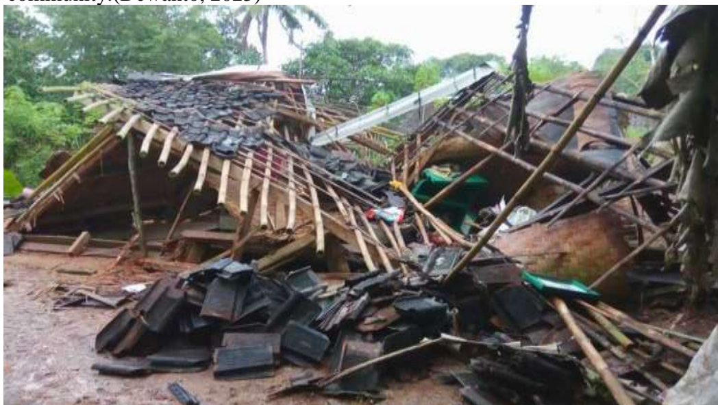
Figure 2. House Destroyed by the Earthquake (Source: Kompas.com)
