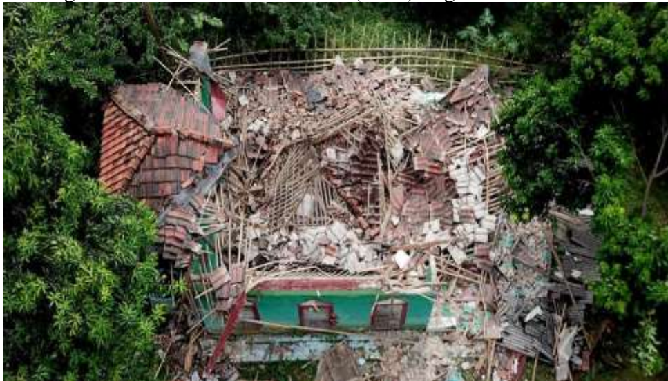
Figure 2: House Damage Caused by the 4.9-magnitude Earthquake (Source: CNN Indonesia)
